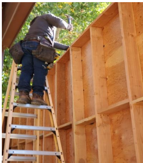
Workman secures wall frame to plywood exterior.
